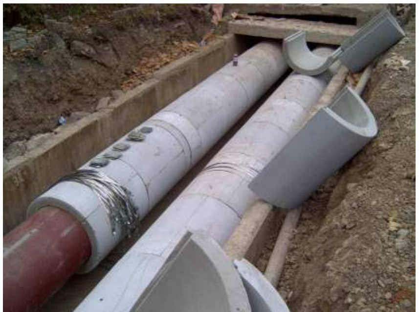
Highly protected: A district heating pipeline, insulated with puren high-temperature-polyurethane-rigid-foam HT; on the left several pipe elements before the installation.
